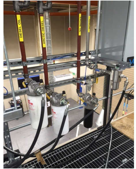
LMP 210 in-line filters and MPS Spin-On for diesel, engine oil, adblue fluid
