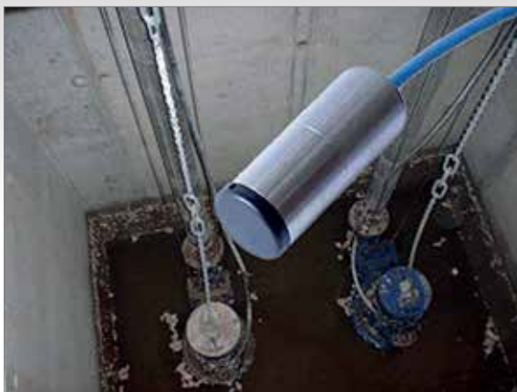
Level sensor ENS Monitors e.g. Wastewater/Water level in a pump shaft
